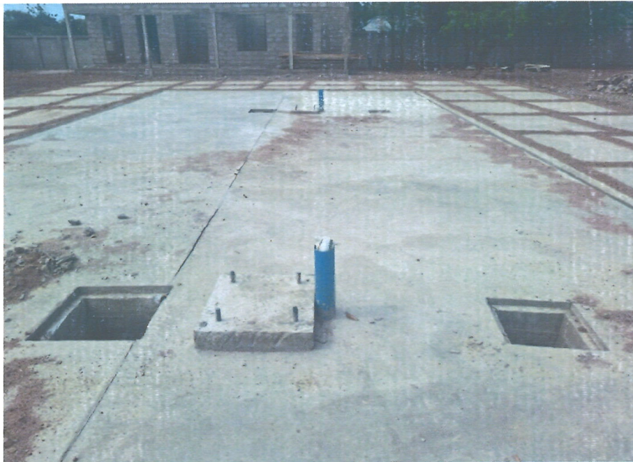
Picture No. 2. Canopy foundation and dispensing area drainage system
